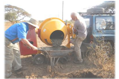
Kenny and Scott working on foundation for brickmaker.
